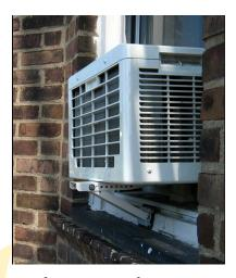
outside air is tree planting to provide shade over your AC unit. There are also products available online when hooked to a water hose will provide a cool mist sprayed around your AC when the compressor comes on. The purpose of both of these ideas is to cool the air some before the compressor goes to work doing additional cooling, lightening the load on your AC, and using less electricity.
